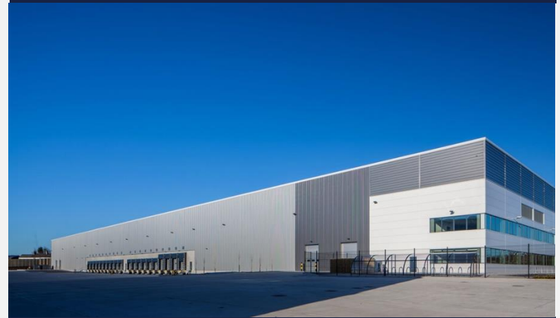
Logistics 225 at Logistics North, Bolton
