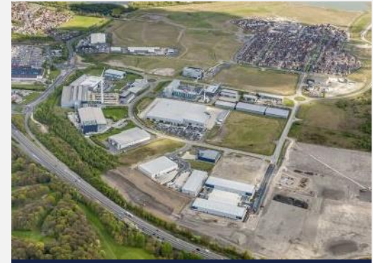
Aerial shot of the Advanced Manufacturing Park, Sheffield J33 M1
