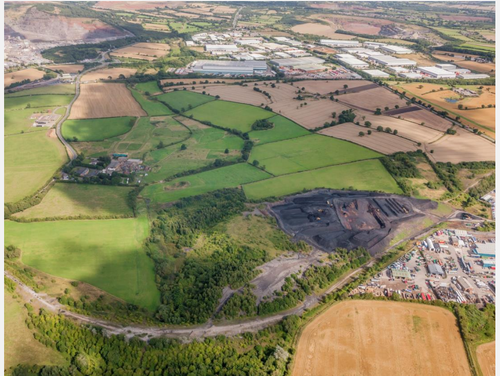
Aerial Photograph of South East Coalville
